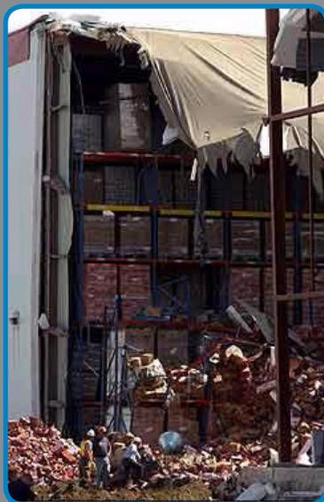
Rack collapse led to surrounding building's collapse
