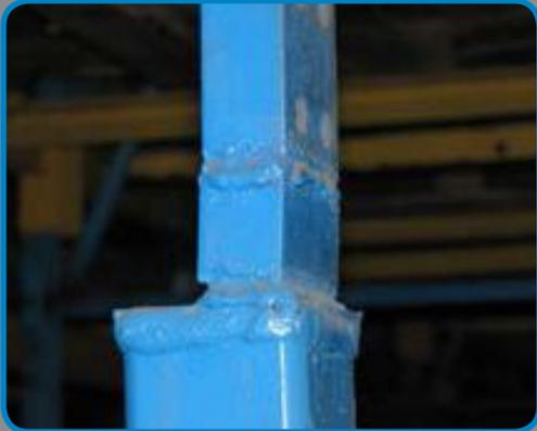
Unsafe Field Welding Repair
